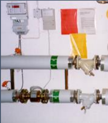
DH metering unit and consumer substation
