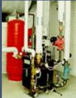
DH metering unit and consumer substation
